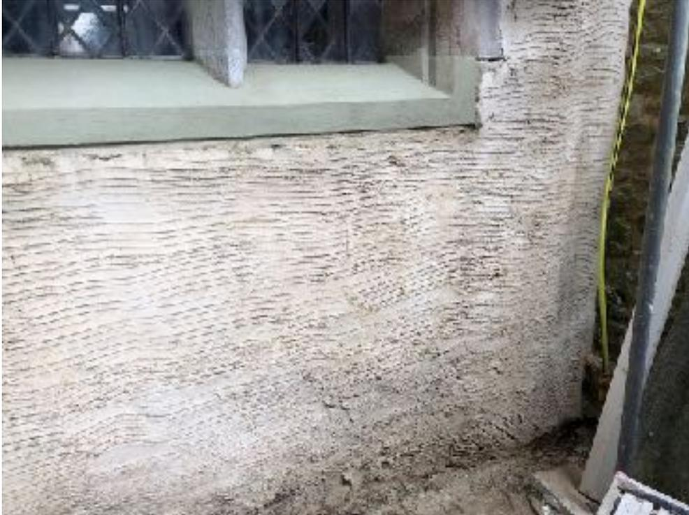
**Plate 7: Scratch coat render applied traditionally at Church of St Mary, Oxted**
